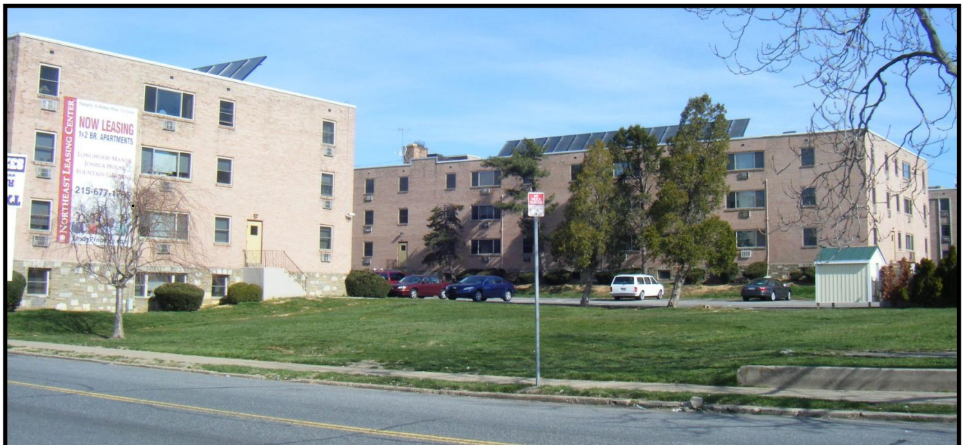
Images courtesy of Rushforth Solar, LLC
