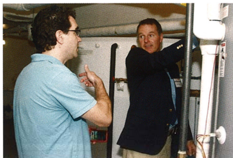
Alan Rushforth has been a passionate proponent of solar hot water, Here he provides a detailed tour of another installation he has designed
